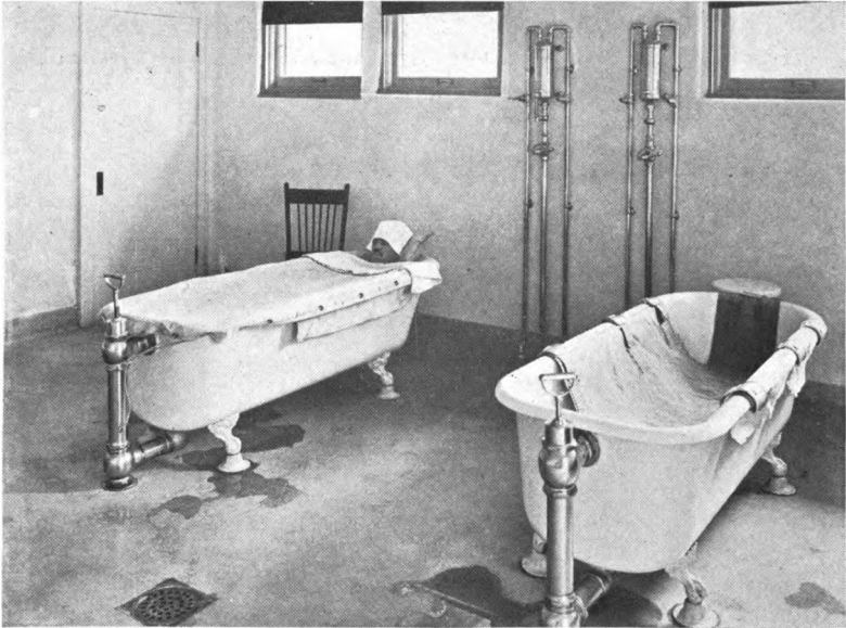
PLATE XX. The continuous flowing bath as installed at the Southern California State Hospital.
